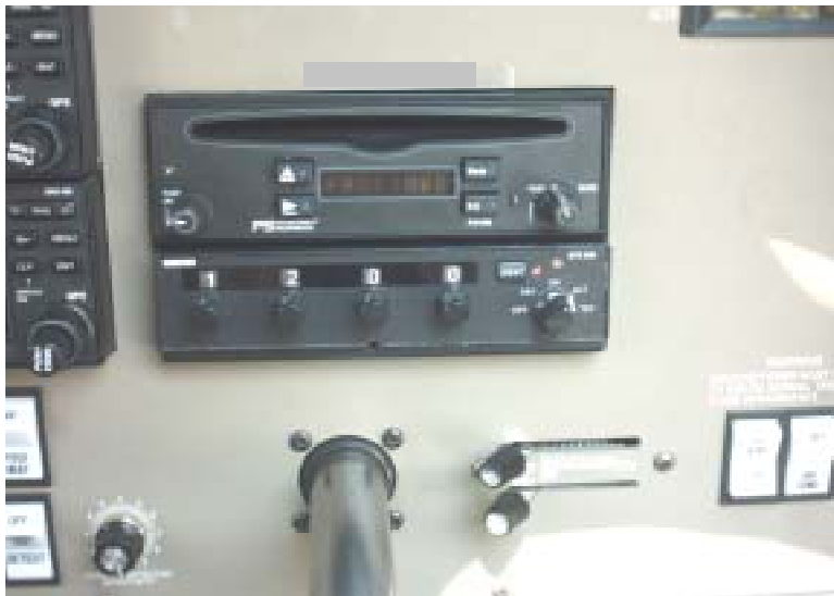
Figure 2-4 Completed panel installation
